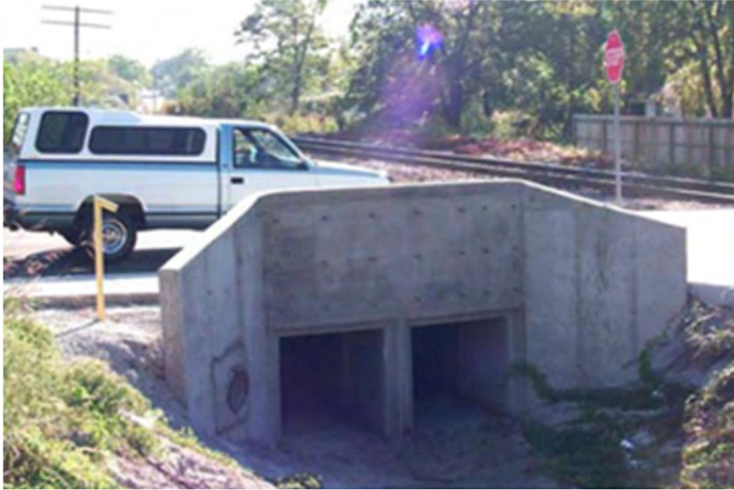
Fig. 30–Walker Box Culvert Bridge
