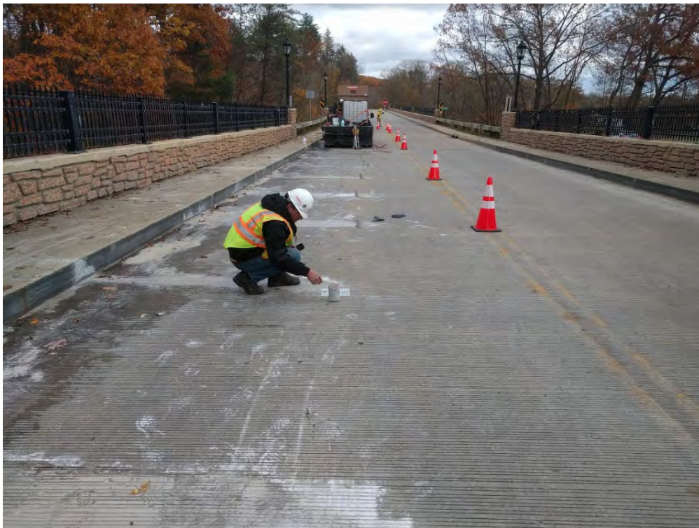
Fig. 17–Coring operation of Cuyahoga Bridge
